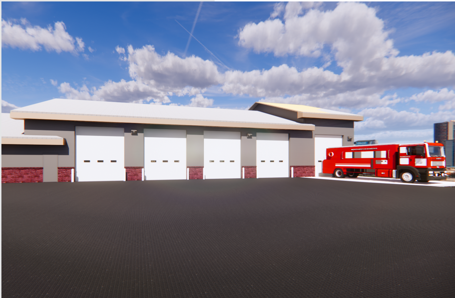
The new addition to the existing fire station.
