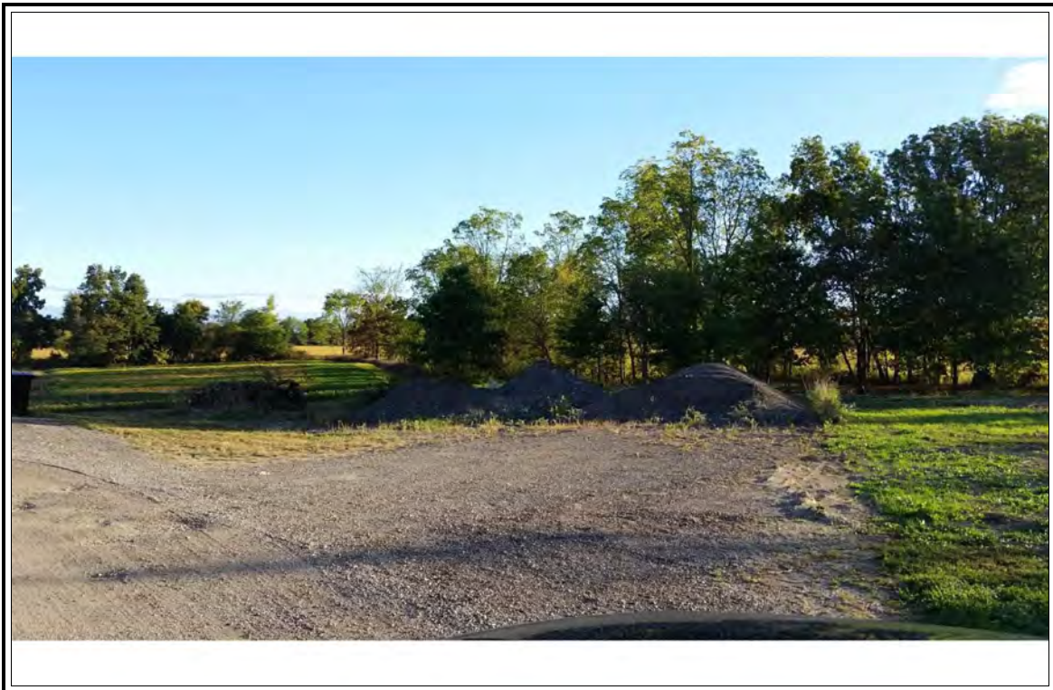
BELOW: Proposed Location of Storage Building Looking NE
