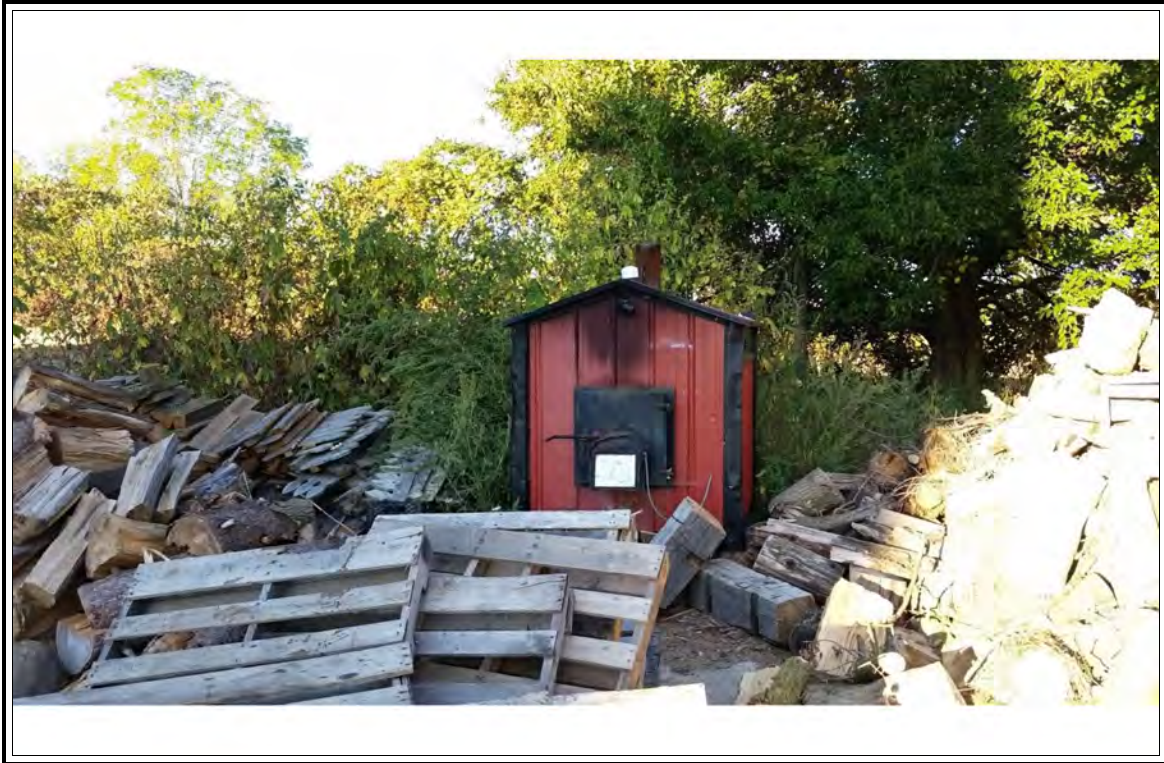
ABOVE: Wood Boiler
