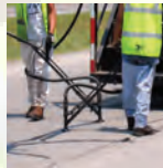
Crack Seal
