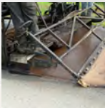
Slurry Seal
